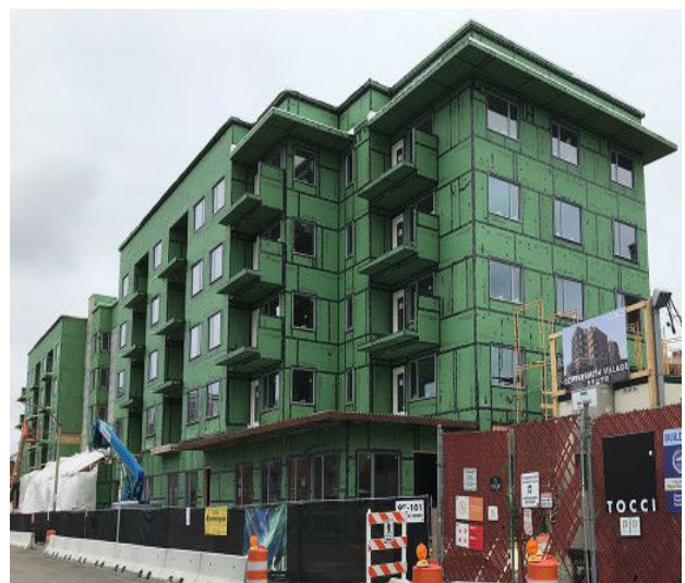
Coppersmith Village nearing completion
