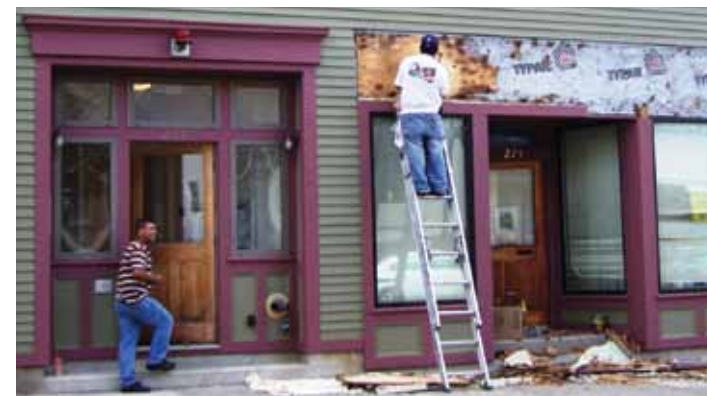
Façade repairs at 277 Meridian Street
